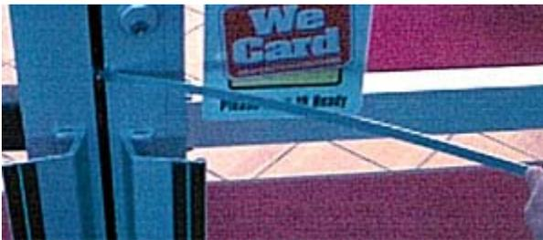
Here we see how the jimmy curves around to touch the door handle, thus fooling the lock into releasing.
